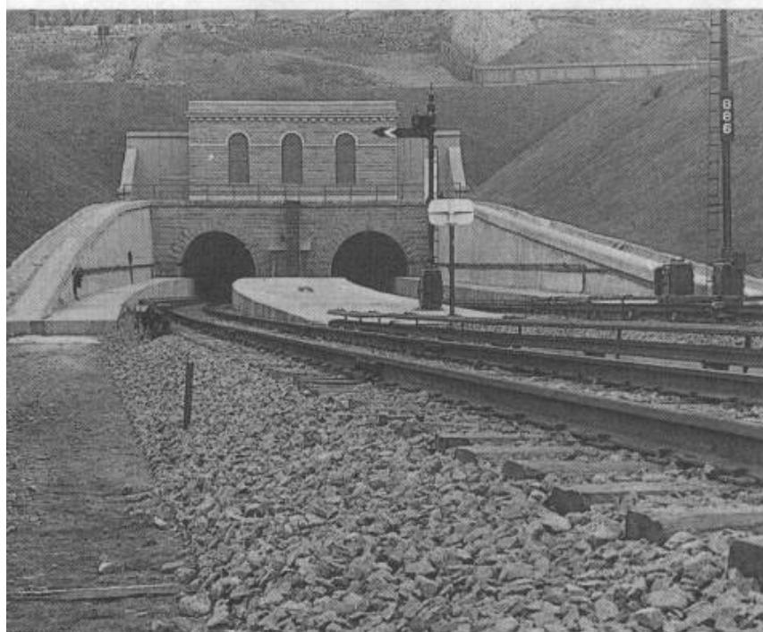
From New Jersey, Pennsy's rails dove under the mighty Hudson through Bergen Portal, described by a contemporary as "a finely proportioned keystone." Photo was taken December 4, 1910, a week after service commenced. Today a highway overpass obstructs the view. (Smithsonian Institution)
